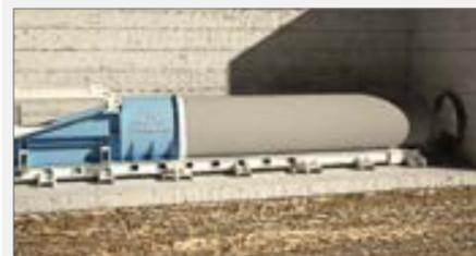
After the auger arrives at the end, the rotation movement stops. The machine is withdrawn by the pipe length, and the other pipe which has an auger in is lowered. By welding,
