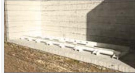
The walking rails of the machine are located in the chimney by a crane, and are located on the base concrete. The walking rails are adjusted according to the drilling axle. The middle axle of the rail should match with the drilling axle.
