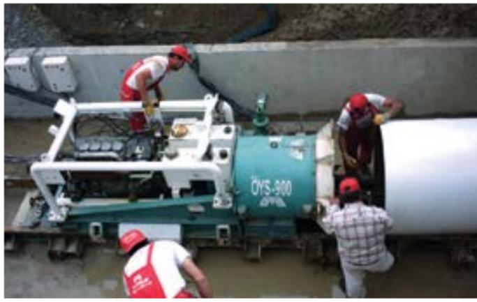
OYS Horizontal Thrust Boring Machines are designed to bore the inevitable need of many public works and construction applications, the coated holes of diameter between 12" and 120".
