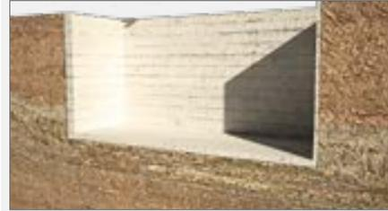
The excavation of the shaft which is convenient for the Project which is prepared according to the sizes of the machine to be used, diameter of the pipe and passing altitude is taken. Then, the formwork is set, the reinforcement is prepared, hip and base concrete is laid. If necessary, the side partition walls are made. Unless there is no danger considering the job safety, the partition walls have no contribution to the horizontal drilling.
