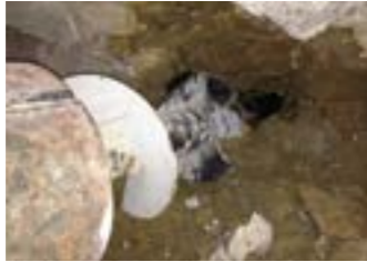
Cutter Head, Auger and Casing While Boring
